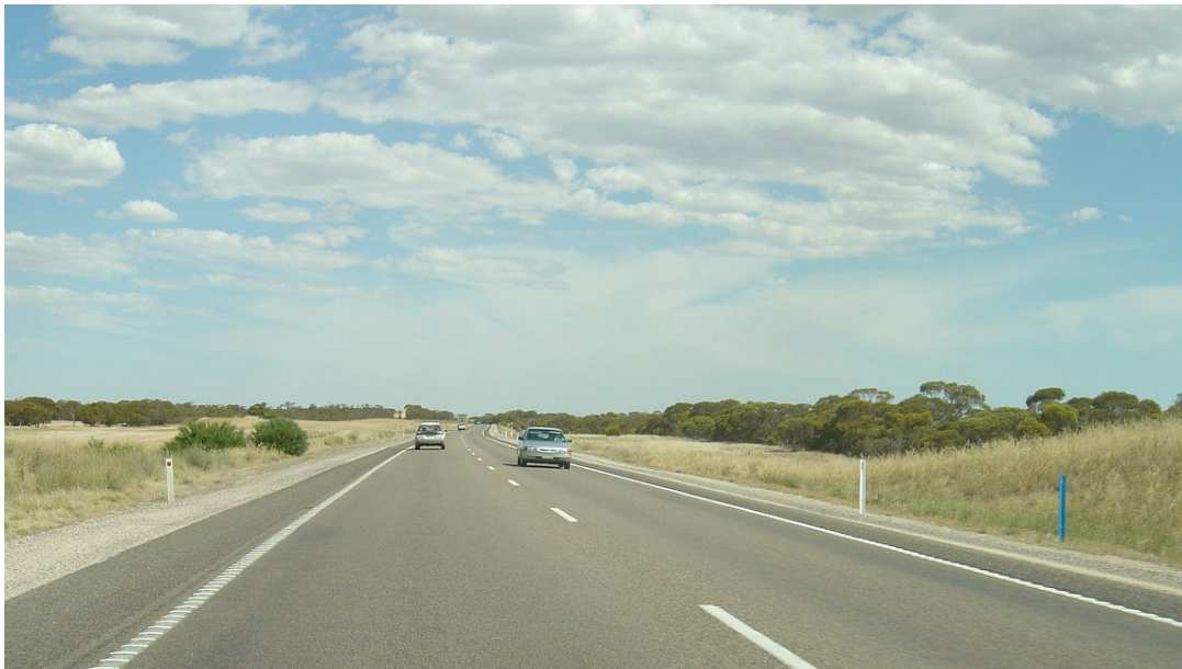
Figure 5.2 Example of thermoplastic ATLM application on the Dukes Highway (J Woolley)
