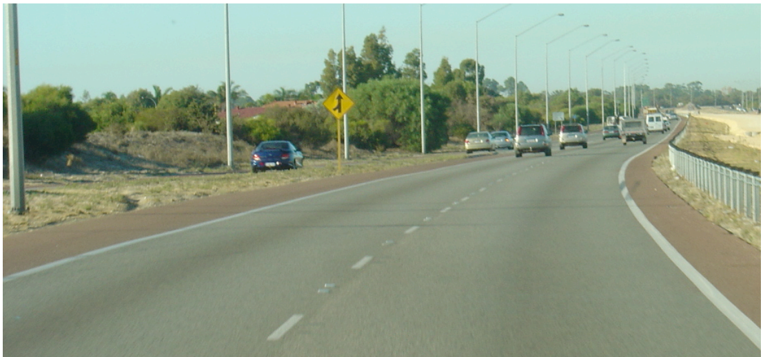
Figure 4.3 Example of contrasting shoulder colours on the Freeway to Mandurah south of Perth (source: J Woolley)
