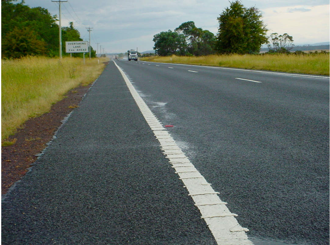
Figure 4.2 Example of ATLM treatment on National Highway One in central Tasmania (source: J Woolley)
