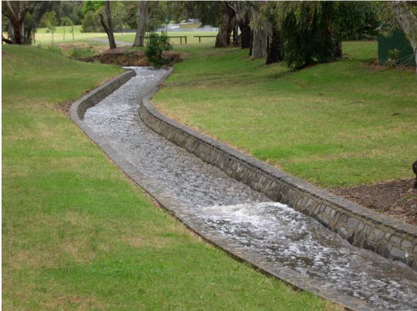
Figure 2.8. Photo of the engineered reach of Fourth Creek. Note the replacement of natural substrates with a cement-slate substrate.
