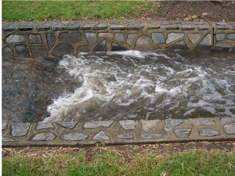
Figure 2.10. Photo of one of three pools within the engineered reach of Fourth Creek.
