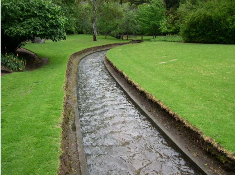
Figure 2.4. Photo of the engineered reach of First Creek. Note the replacement of natural substrates with a cement-rock substrate and the increased level of bank erosion.
