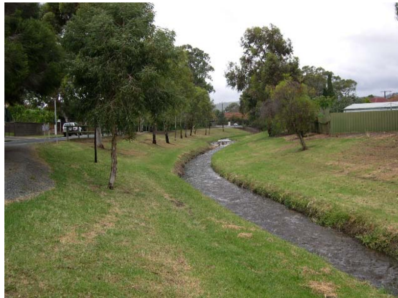
Figure 2.7. Photo of the degraded reach of Fourth Creek. Note the increased level of stream bank erosion and the channelised structure of the reach.
