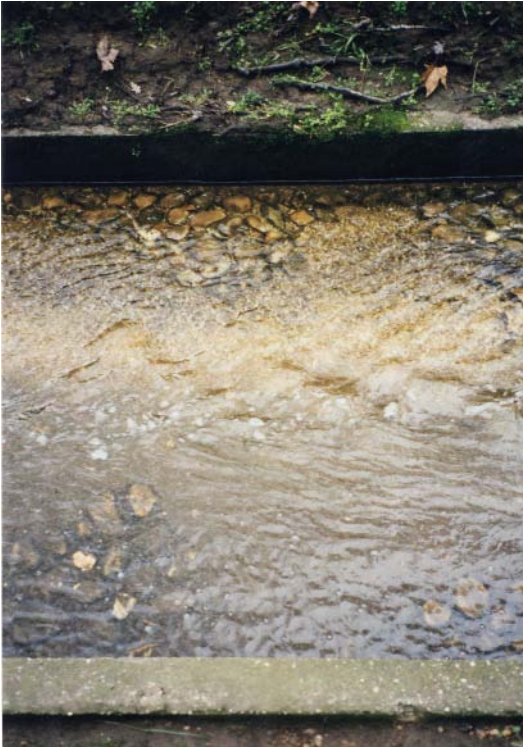
Figure 2.5. Photo of the stream bed (aerial view) of the engineered reach of First Creek. Note the replacement of natural substrates with a cement-rock substrate.
