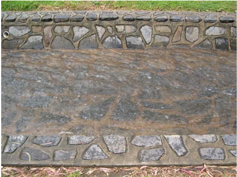
Figure 2.9. Photo of the stream bed (aerial view) of the engineered reach of Fourth Creek. Note the replacement of natural substrates with a cement-slate substrate.
