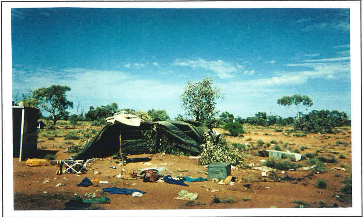
FIGURE 27: Wiltja constructed of various materials including vegetation, tarpaulins and reinforcing mesh. Note: galvanised tucker box in the foreground to secure foodstuffs.
