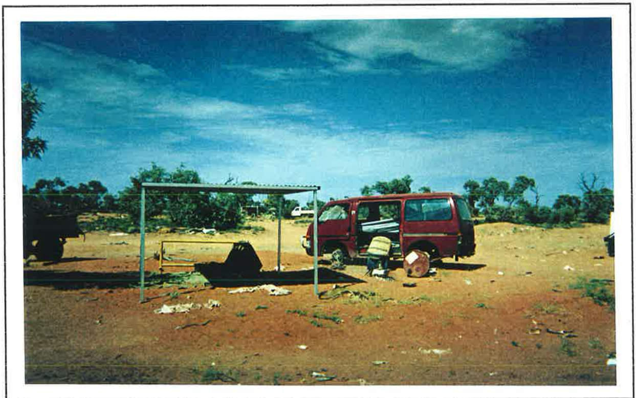
FIGURE 28 : Car body being used as housing in conjunction with community-built shelter. In this example, ablutions and other services are available at the adjoining house.
