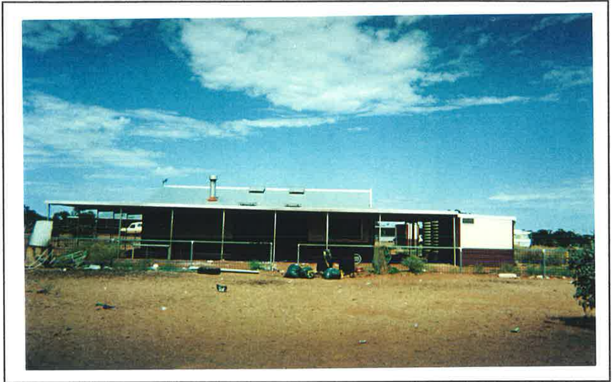
FIGURE 31 : Nomadic housing (Model H3-35) constructed in 1997. Features include three lockable bedrooms, separate kitchen and living area incorporating earthen floor. Ablution/laundry block is located to the left and a pit toilet is located at the rear of the property.
