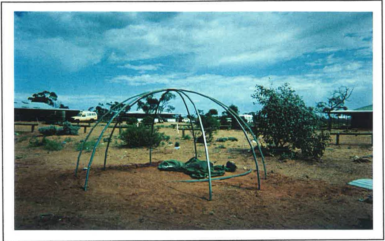
FIGURE 33 : Larger wiltja frame in place at Oak Valley. No damage to frames was observed. These larger frames may be difficult for elderly residents to carry and construct. In this instance the tarpaulin was torn.
