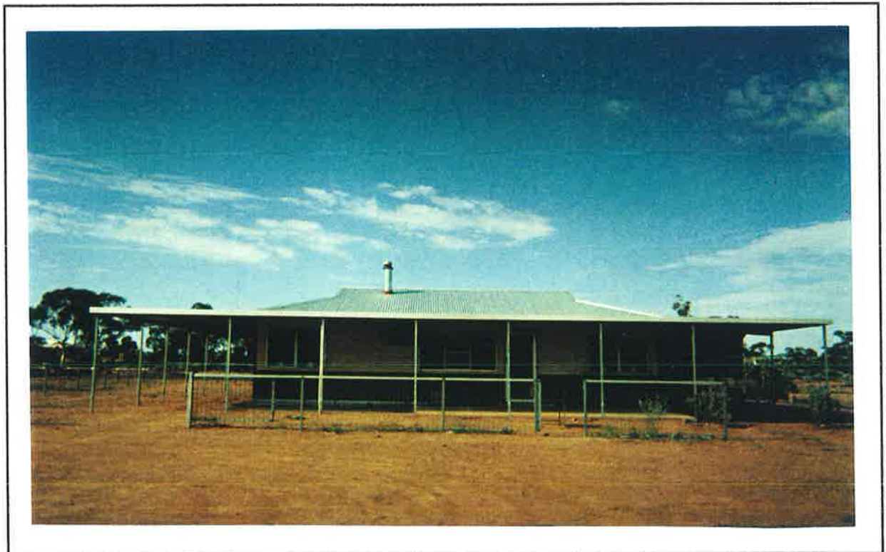
FIGURE 32 : Nomadic Housing at Oak Valley (Model H3-29). Ablutions/laundry block adjoins rear verandah. Pit toilet is located at the rear of the property. All fencing is constructed of reinforcing mesh.
