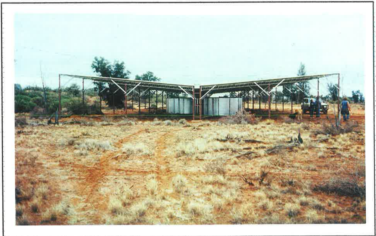
FIGURE 24: Water shed. This example is located along the Aquitaine Road south of Oak Valley. The water shed collects rain from isolated thunderstorms and supplies shelter to people travelling between Oak Valley and Yalata. source : Aboriginal Housing Authority
