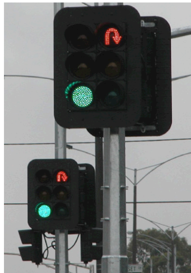
Figure 2 Example of U-turn signal phasing in use in Melbourne (photo courtesy of Akcelik and Associates, Melbourne)
