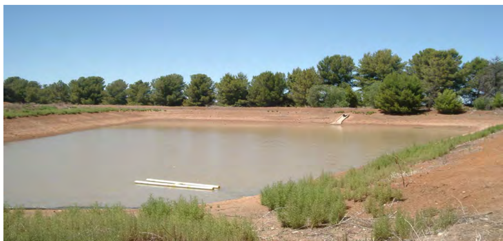
Figure 186 Snowtown - Community Stormwater Dam (Rabone 2003)
