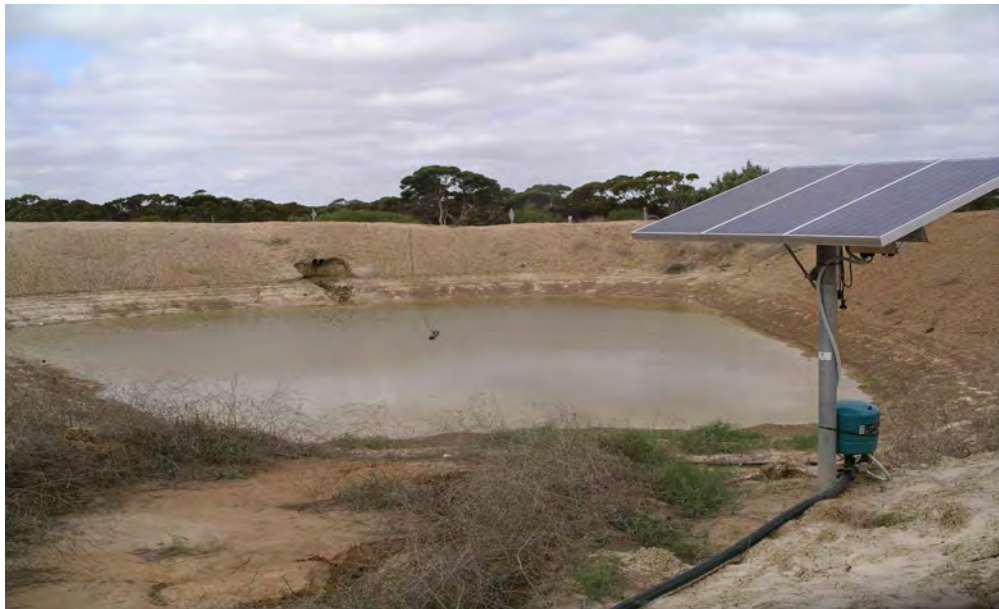
Figure 154 Lock – Stage 2a Community Stormwater Dam (Rabone 2006)
