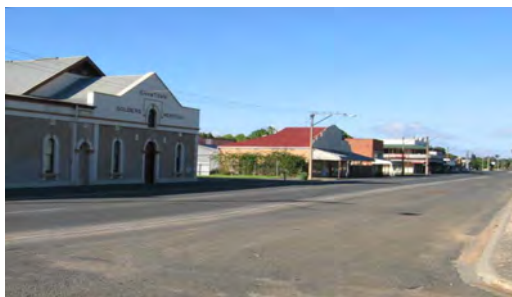
Railway Terrace East
