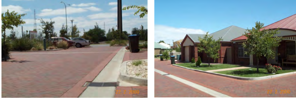
Figure 160 New Haven Village – Streetscape & Drains (Rabone 2000)
