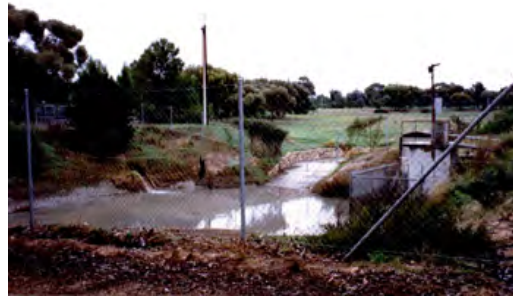
Stormwater Pumping Pond
