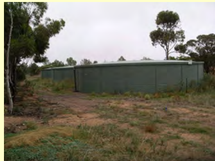
Irrigation Storage Tanks
