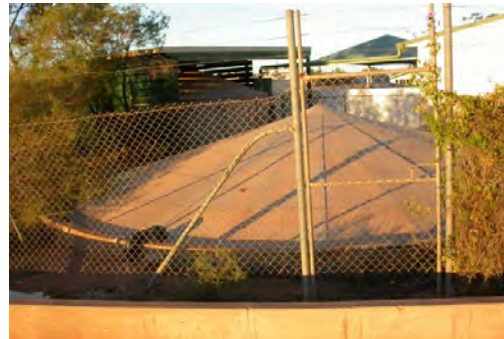
School Runoff Storage
