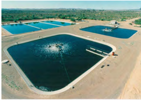
Treatment Plant (ETSA 1993)
