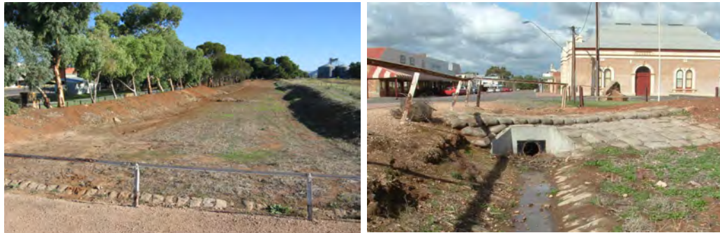
Retention Basin (Upstream)
