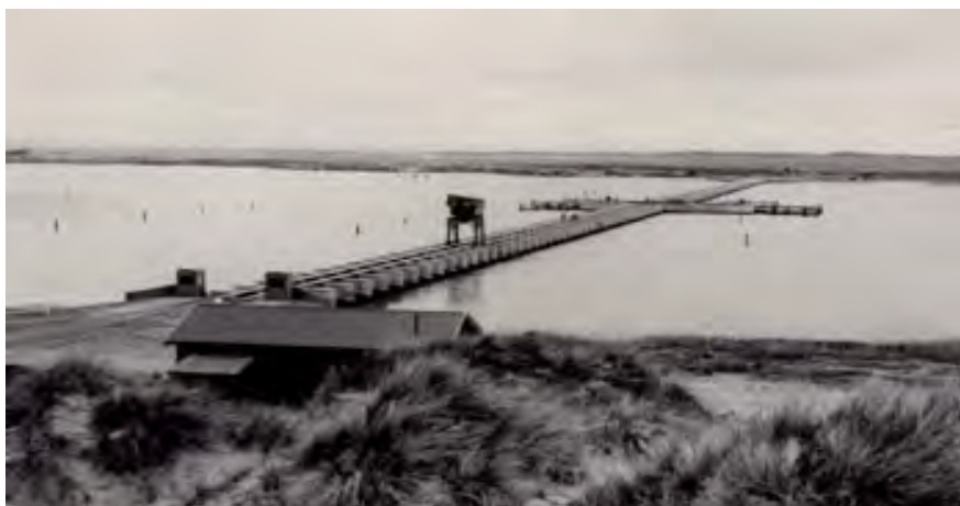
Figure 228 General View of Goolwa Barrage (SA Water Photo Catalogue)
