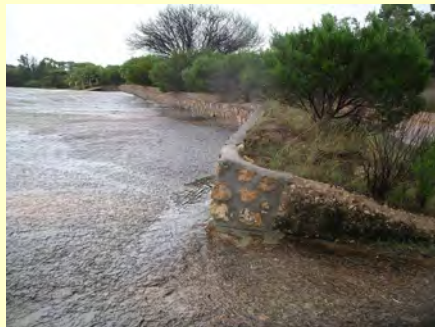
Low walls around base of rock
