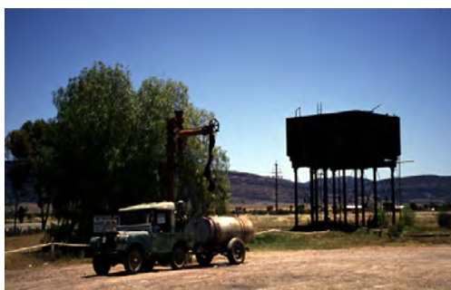
Elevated Tank & Standpipe
