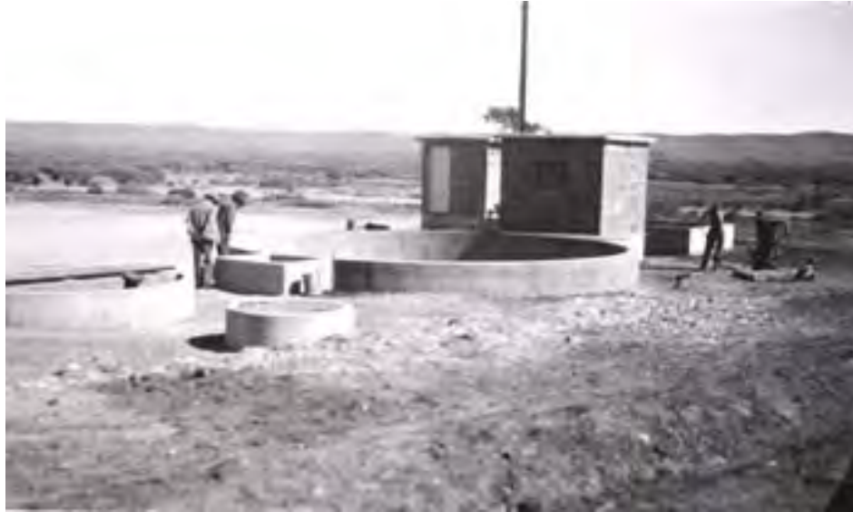
Figure 233 Leigh Creek Sewage Treatment Plant, 1946 (SA Water Photo)
