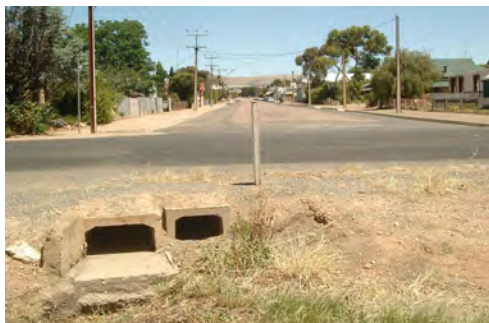
Progressively Sealed between Kerbs
