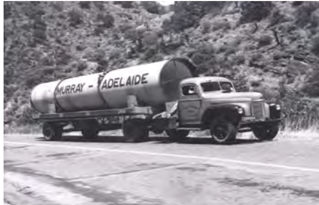
Figure 229 MAPL - First pipe en-route to Mannum (SA Water Photo)
