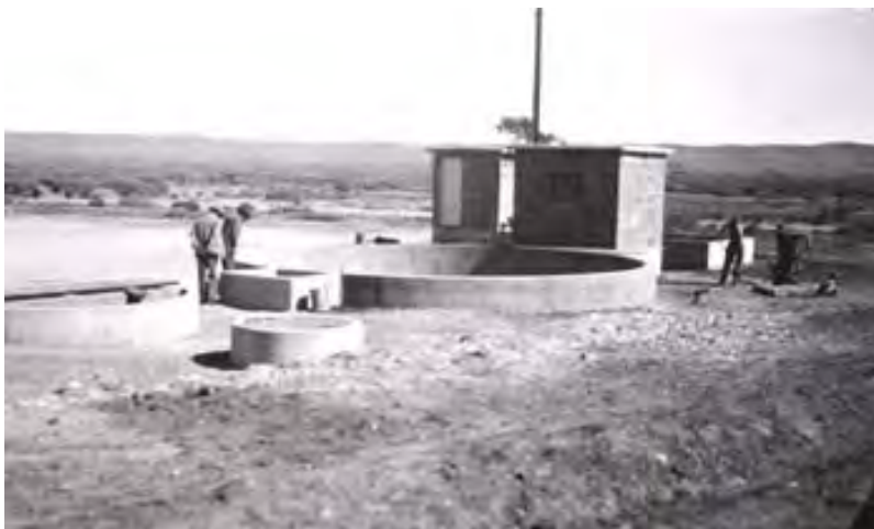
Figure 135 Leigh Creek – Wastewater Treatment Plant 1946 (SA Water)
