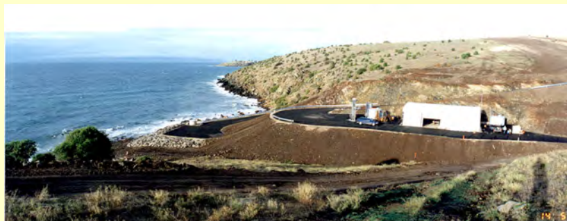
Figure 54 Penneshaw Desalination Plant: Site after construction
