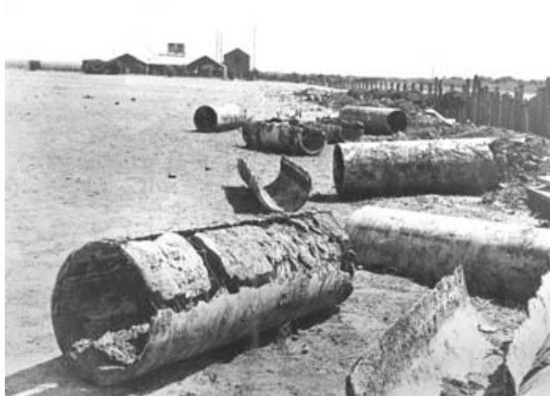
Figure 232 Deterioration of Sewers, Islington 1936 (SA Water Photo Collection)
