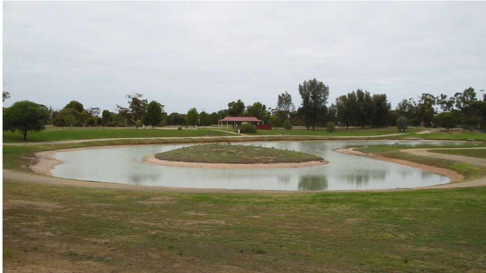
Figure 131 Lameroo - Stormwater Lake & Emergency Storage (Broughill)
