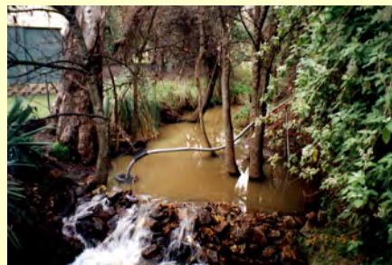
Brown Hill Creek Intake
