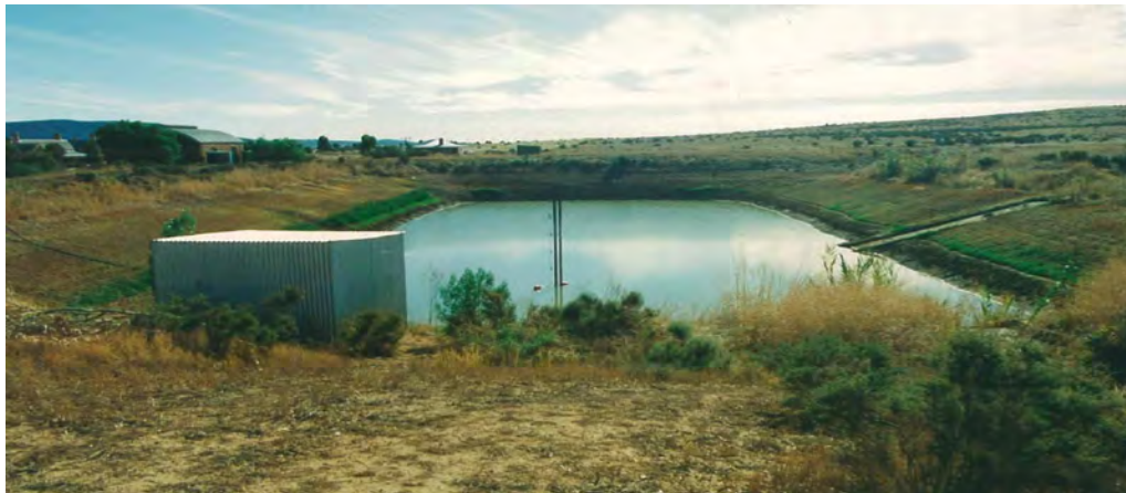
Figure 125 Hawker Community Stormwater Dam (Rabone 1996)
