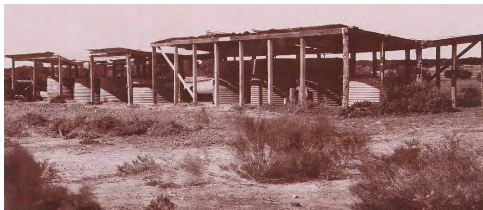
Figure 227 Early Water Supply: The Lady Kinard Shed Tank (EWS 1987)
