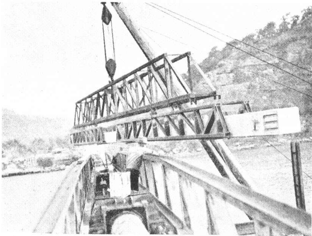
LIFTING TACKLE FOR CONCRETE PILES.
