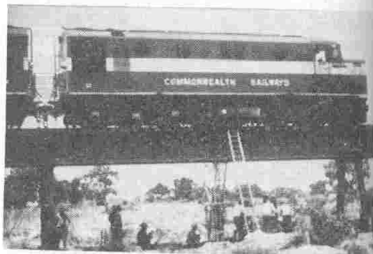
Showing our faith in the bridge!
