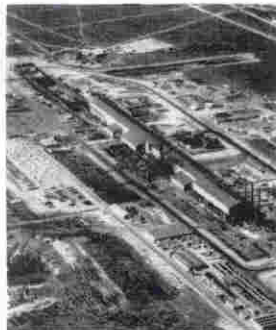
BHP's Rolling Mills. ASEA switchgear controls the entire finishing end.
