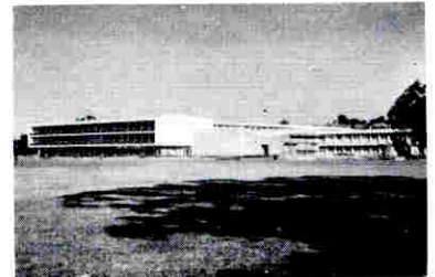
THE NEW PERTH ENGINEERING BUILDING OPEN- ED AT THE BE- GINNING OF THE SYMPOSIUM
