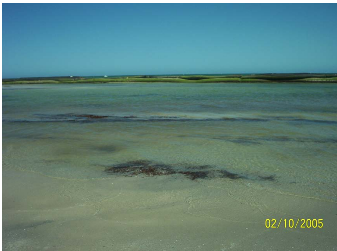
Figure 46 Point Malcolm geotextile breakwater seen from shore at low tide.
