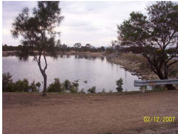
Figure 49 West Lakes/ Port River barrier on left.
