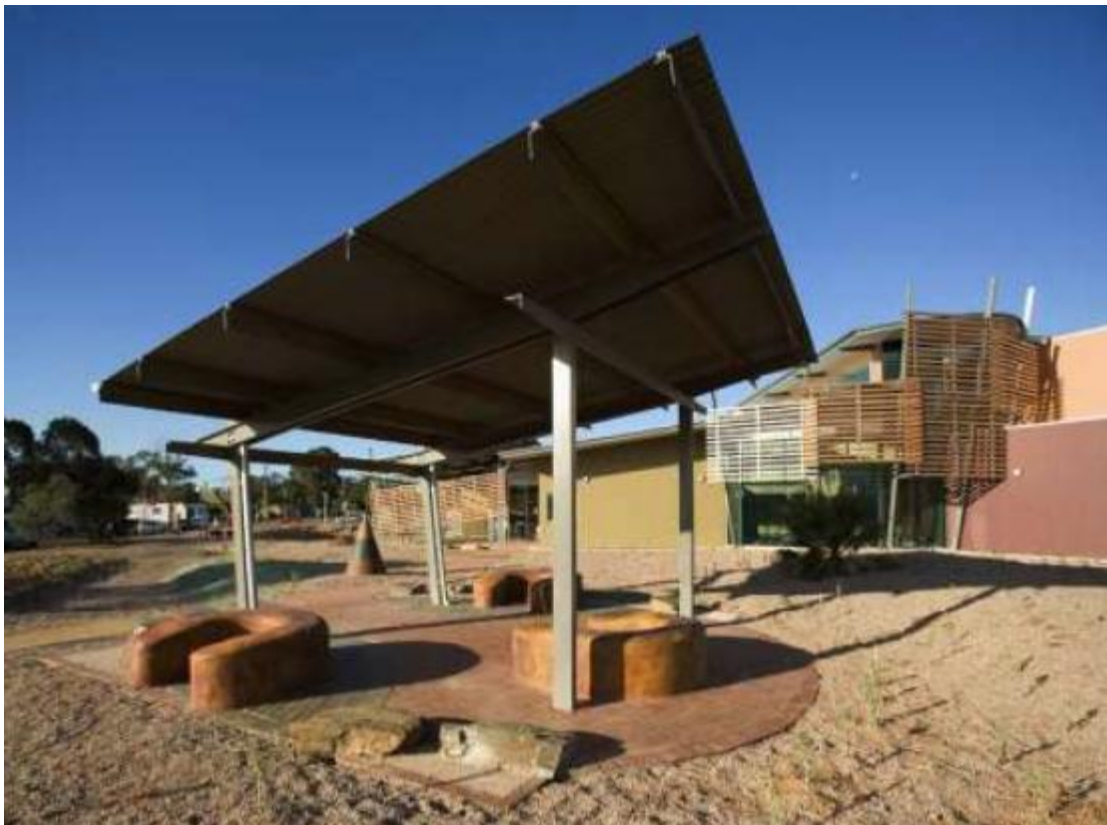
Figure 46: Port Augusta Courts Complex (Architect: Denis Harrison, Government of South Australia). The external areas designed around the courts complex provide discrete waiting and gathering areas for traditionally oriented Aboriginal people. Note: Photograph taken prior to vegetation being planted (Photographs: Ben Wrigley).
