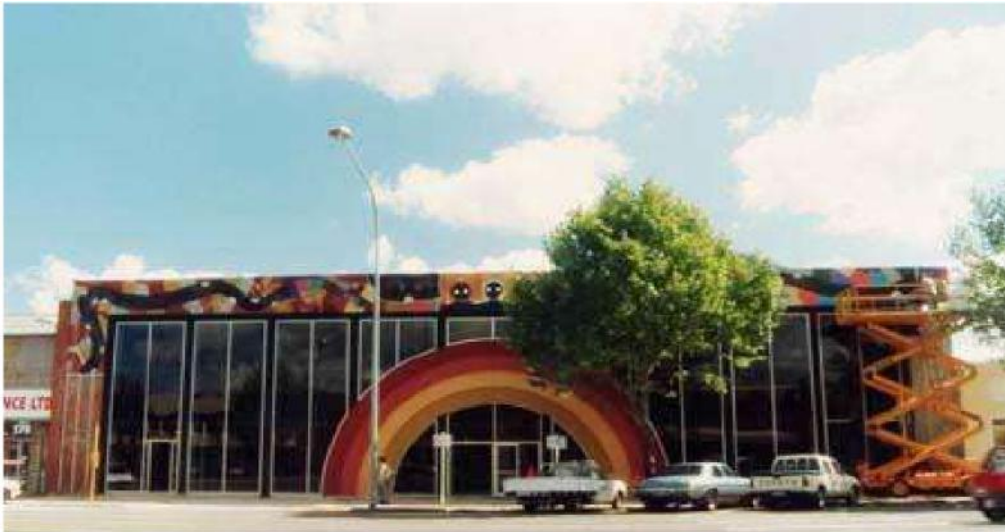
Figure 51: Nunkuwarnin Yuntji, Adelaide. The frontage of the building (a former retail showroom) has no signs indicating it is a community controlled health centre, but instead is decorated in specific colours and layered with symbols and icons (Photograph: Grant).
