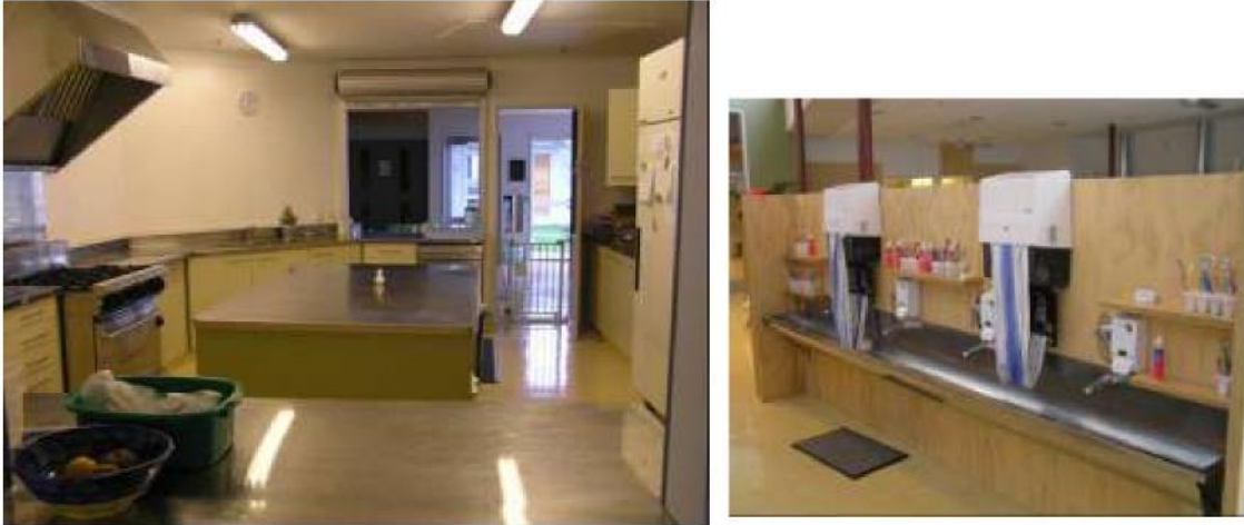
Figure 54: Mana Tamariki, Palmerston North (New Zealand) (Architects: Tennent and Brown) kitchen and alcove for hand washing next to kitchen (Photographs: Ministry of Education New Zealand, 2006).
