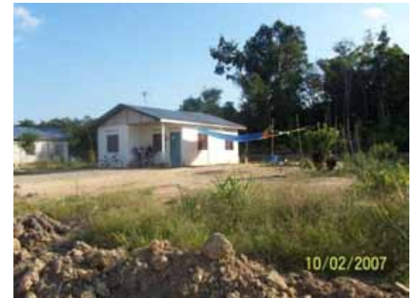
Examples of new houses from the PPRT scheme at Kg Jelawat
