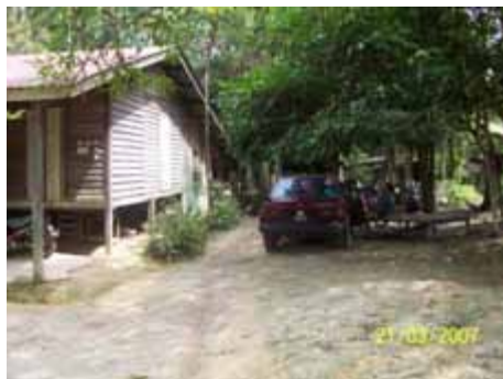
House No 13: View of the side yard Date Photo Taken: March 21 st ,2007
