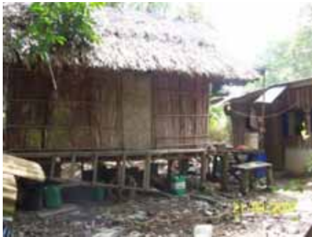
House No 14: the front facade of the house Date Photo Taken: March 21st,2007
