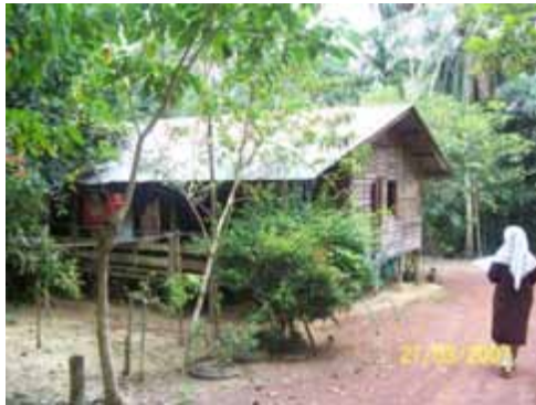
House No 18: View from the driveway towards the house Date Photo Taken: March 21 st ,2007
