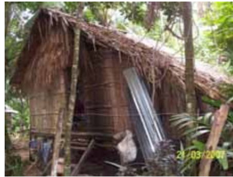
House No 12b: the front facade of the house Date Photo Taken: March 21 st ,2007
