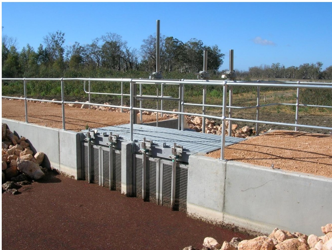
Figure 1.2. Carp screen located at Webster's Lagoon, north-west Victoria.
