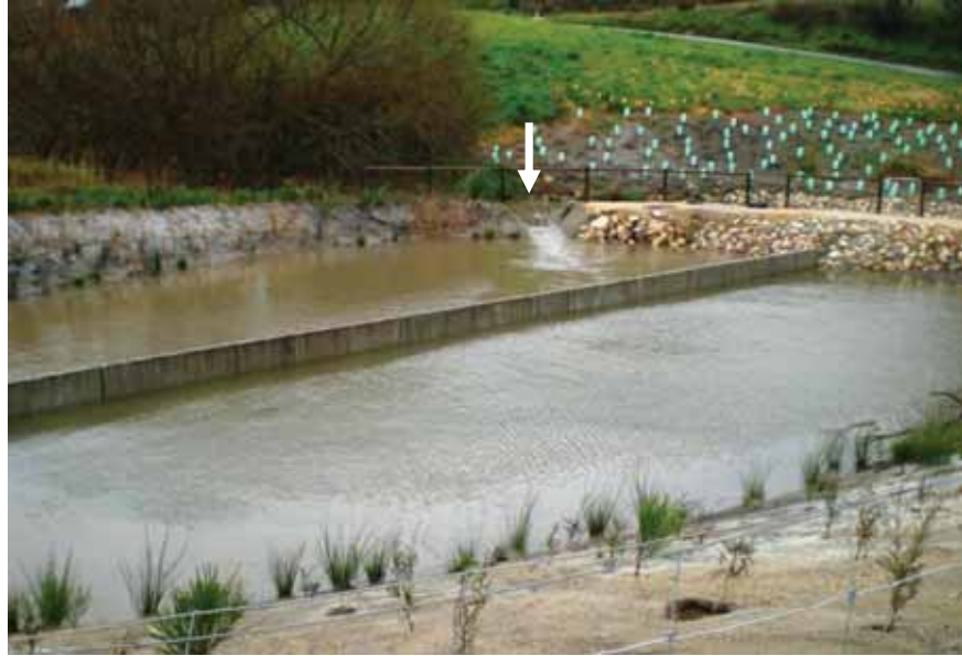
Figure 2.6: Photo of the offline Brookes Bridge sedimentation basin. Note that arrow represent the inflow of water through the sedimentation basin from the upper Cox Creek sub-catchment.
