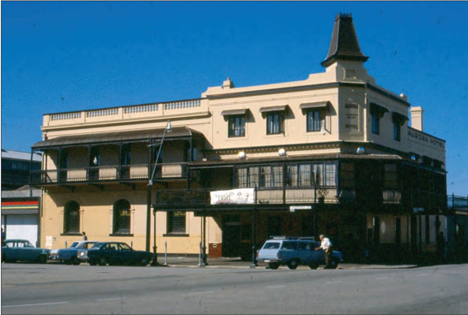
Figure 35: Aurora Hotel, Hindmarsh Square, before demolition
