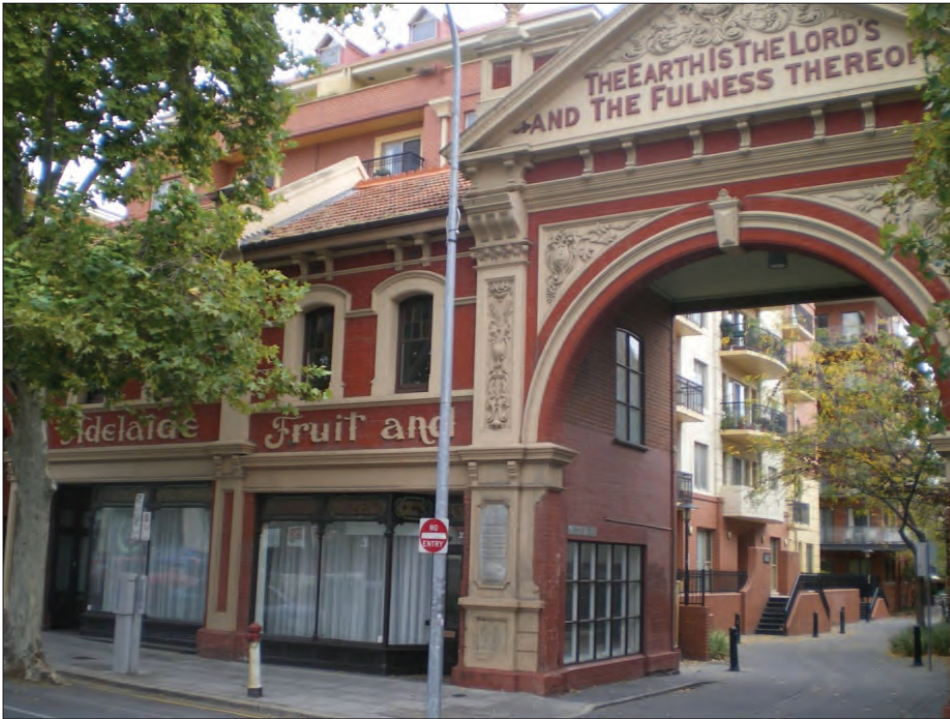
Figure 40: The redeveloped East End Markets (Heritage façade retained with new residential development behind)
