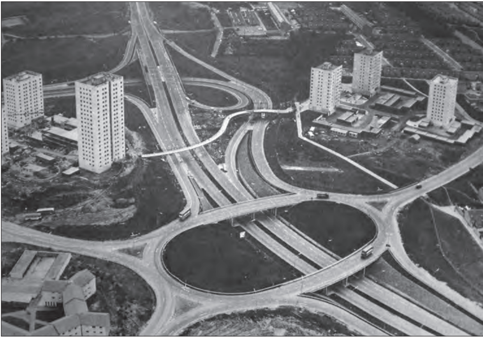
Figure 17: Tower blocks and motorways in Cumbernauld New Town
