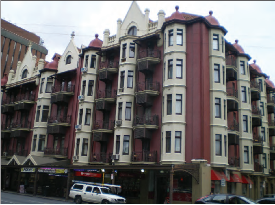
Figure 31: Ruthven Mansions after restoration
