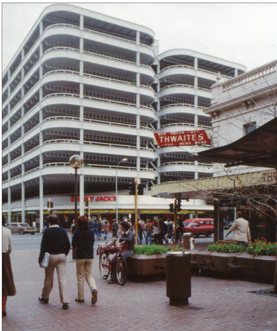
Figure 22: The demountable Rundle Mall Car Park
