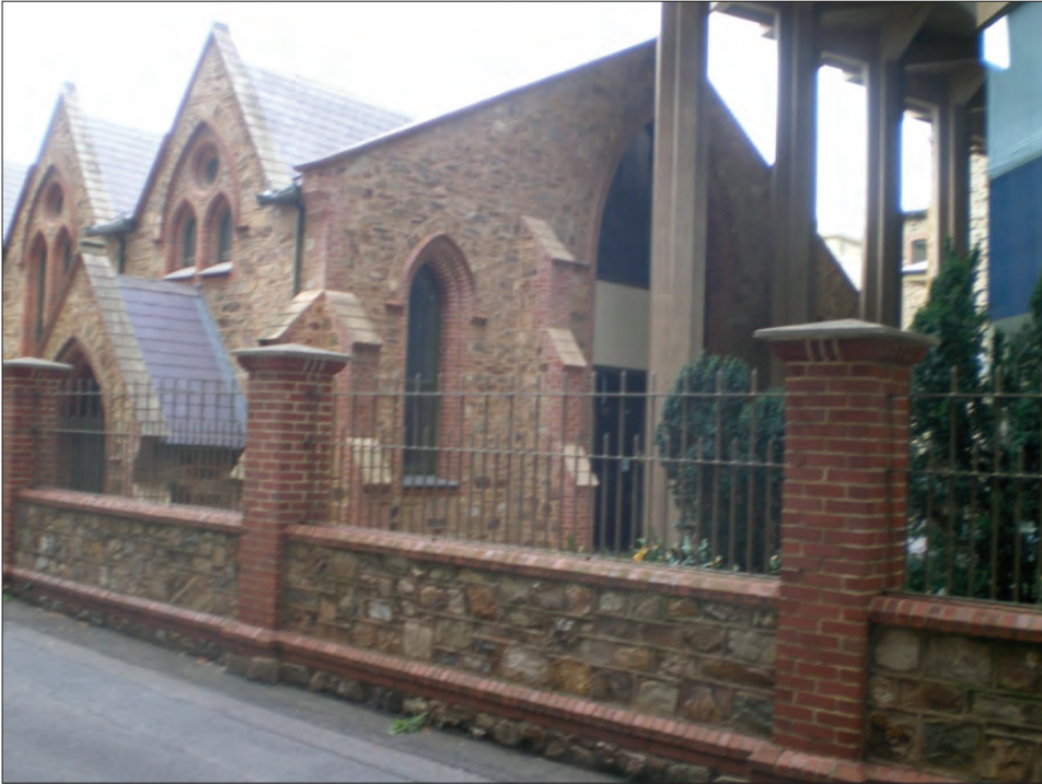
Figure 33: The new northern wall of the restored Old Methodist Meeting Hall
