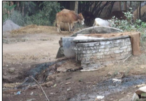
Figure 6.13: An unrepaired Government built (non Grameen Shakti) biogas plant.
