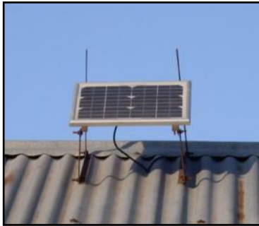
Figures 4.4 and 4.5: Grameen Shakti solar home system. A small solar home system panel on a customer’s roof (left); a customer standing next to the charge controller above and the battery below (right). Note: Photos from author, permission granted for publication by customer pictured, Bangladesh village 2008.
