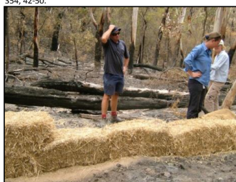
Figure 3: Installing sediment barrier traps
