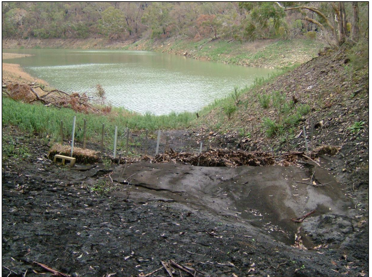
Hay bale sediment barrier near the reservoir four months after the Mount Bold wildfire
