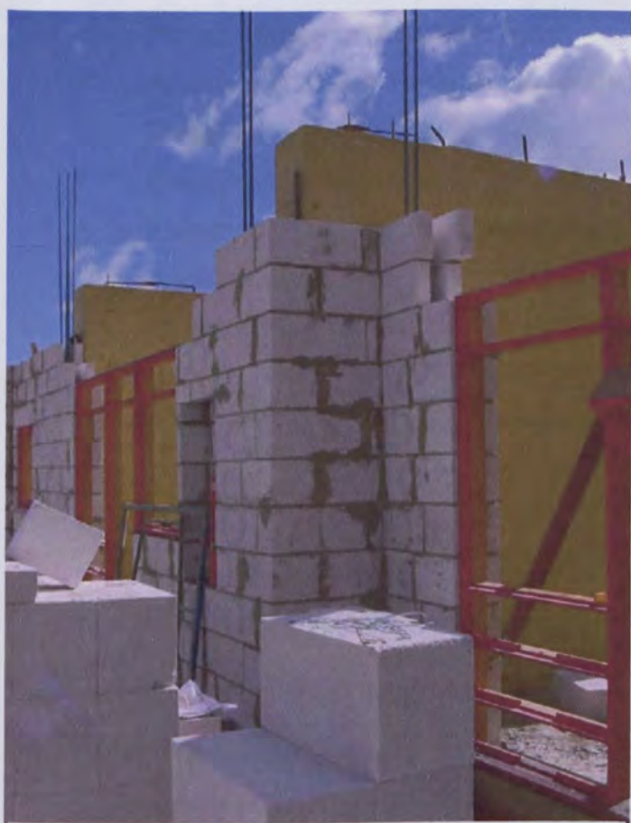
FIGURE 164: Stage 1, South side under construction. (Photo by author)
