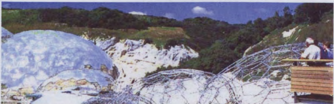
FIGURE 43: Eden Project domes under construction. (Source: World Architecture Pawley 2001)
