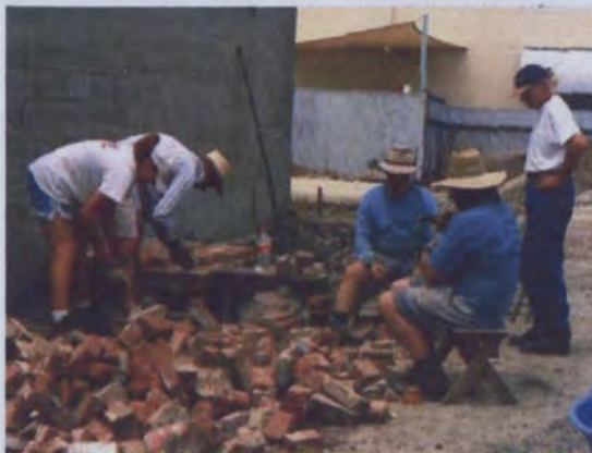
FIGURE 163: Volunteers cleaning bricks for decorative paving and fossicking for ceramics and bottles. (Photo by author)
