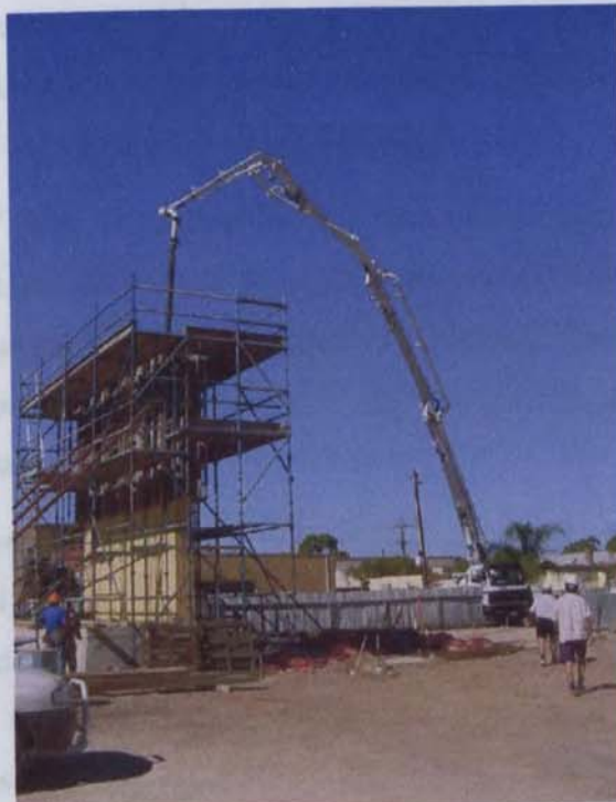
FIGURE 178: Pouring the first 'earthcrete' wall. (Photo by author)
