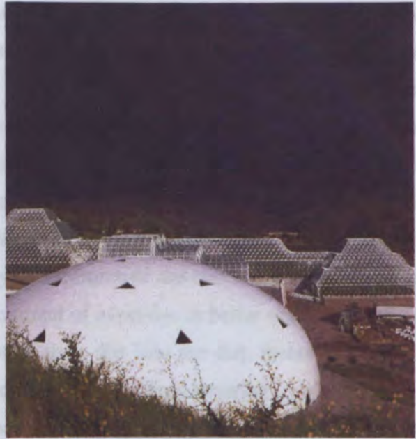
FIGURE 17: Biosphere 2, Oracle, Arizona. Dome of pressure equalisation 'lung' in foreground. (Source: Allen 1991 p.65)
