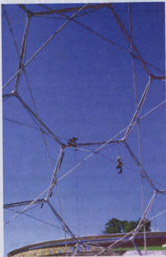
FIGURE 12: Eden Project domes under construction. (Source: World Architecture , Pawley 2001)
