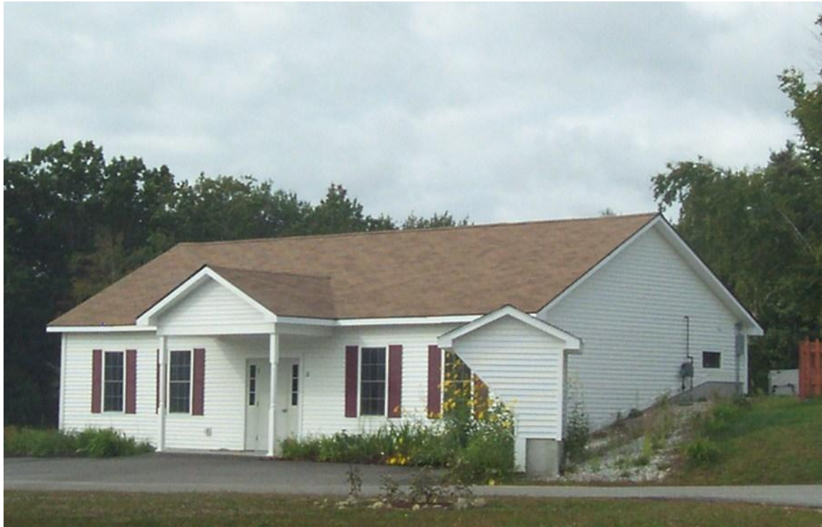
Figure 6.8 Pepperidge Woods Cooperative’s community house. The structure at the front (foreground, right) contains the community’s mail boxes. Photo: The author
