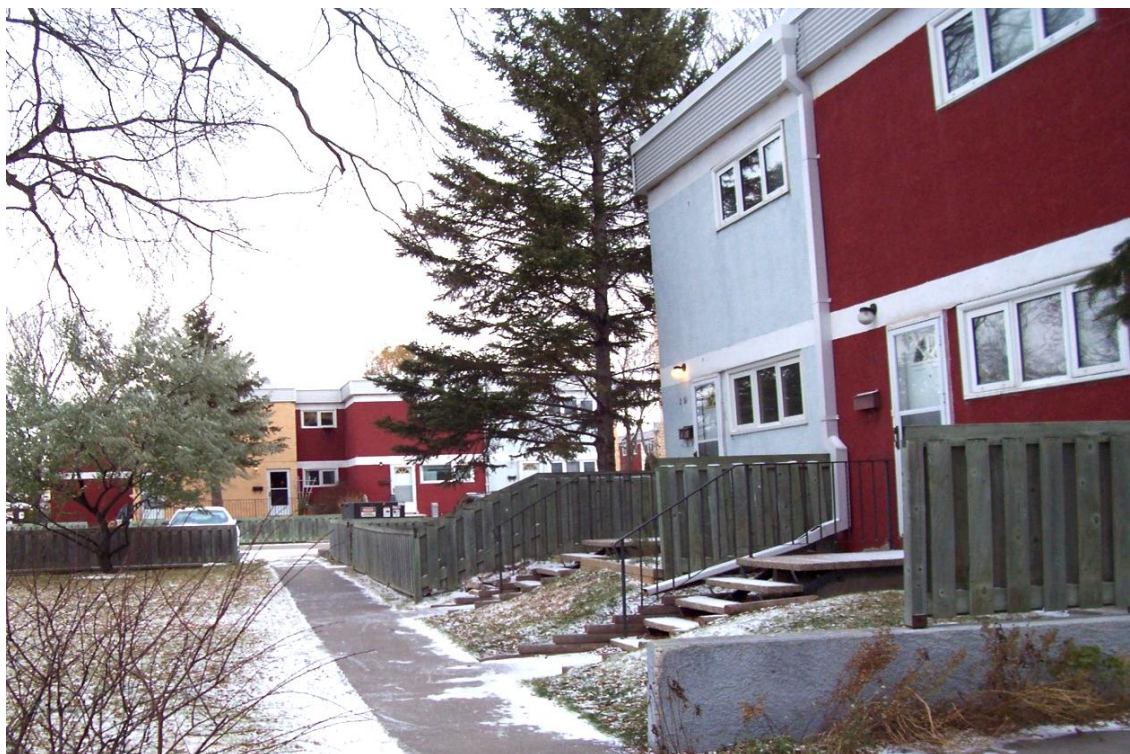
Figure 7.3 Willow Park Cooperative's design features a network of courtyards. Photo: The author
