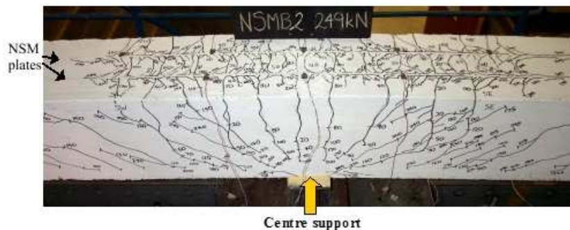
Fig. 5 Debonding of NSM plates
