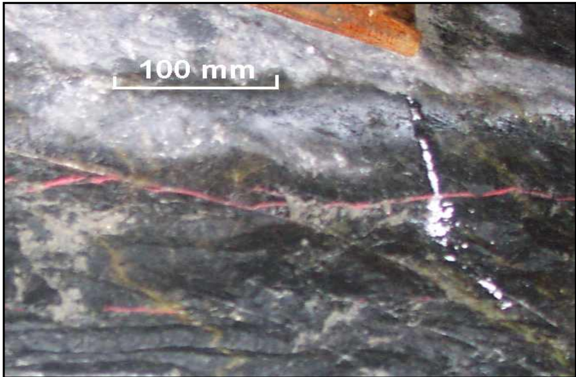
Figure 4. Hydraulic fracture offsetting along a natural fracture. This photo was taken after mining of an access decline at Northparkes E26 mine. The hydraulic fracture growth was defined by using a red plastic proppant. The injected water contained fluorescein to serve as a fracture fluid marker. After van As and Jeffrey (2002)
