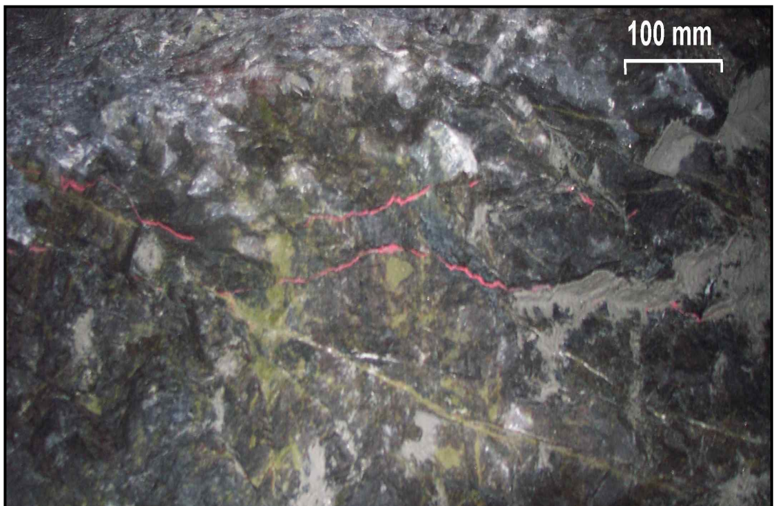
Figure 5. Hydraulic fracture that consists of two parallel branches. This photo was taken after mining of an access decline at Northparkes E26 mine. The hydraulic fracture growth was defined by using a red plastic proppant. The injected water contained fluorescein to serve as a fracture fluid marker. After van As and Jeffrey (2002)
