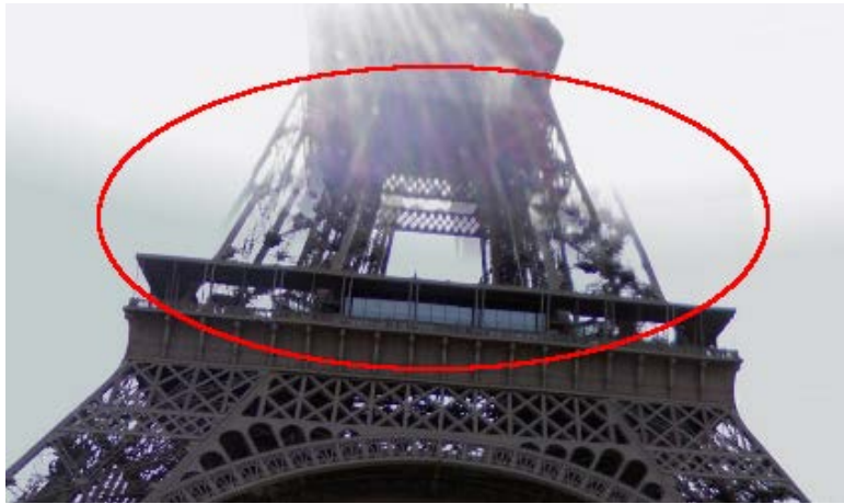
Figure 1.4: A magnified (and cropped) view of Fig. 1.2 that shows some of the artifact errors (circled in red) caused by failed post-processing routines in image stitching. This problem is probably because most of the images used in Google's street view are obtained with cameras mounted on vehicles, undergoing translational motions.
